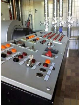
Thirty years ago, operator stations consisted of indicators, push-buttons, possibly a recorder, all mounted in the door of a large enclosure or on the face of a pedestal enclosure. Inside the box was the PLC, and each of the components of the operator station had to be hard-wired together by hand. Each of the terminations and each of the components was a single point of failure just waiting to happen and the cost of producing each operator station was very high.
